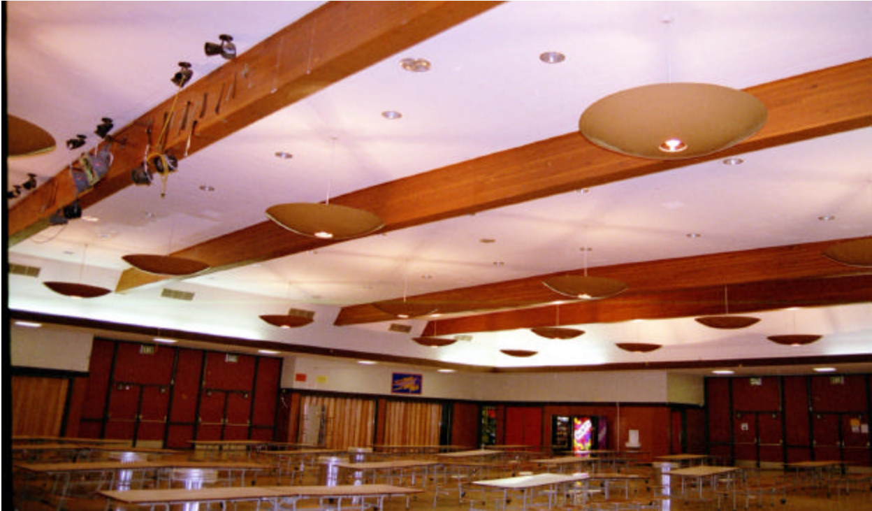
Figure 11: Roof Framing of Multi-Purpose Room
