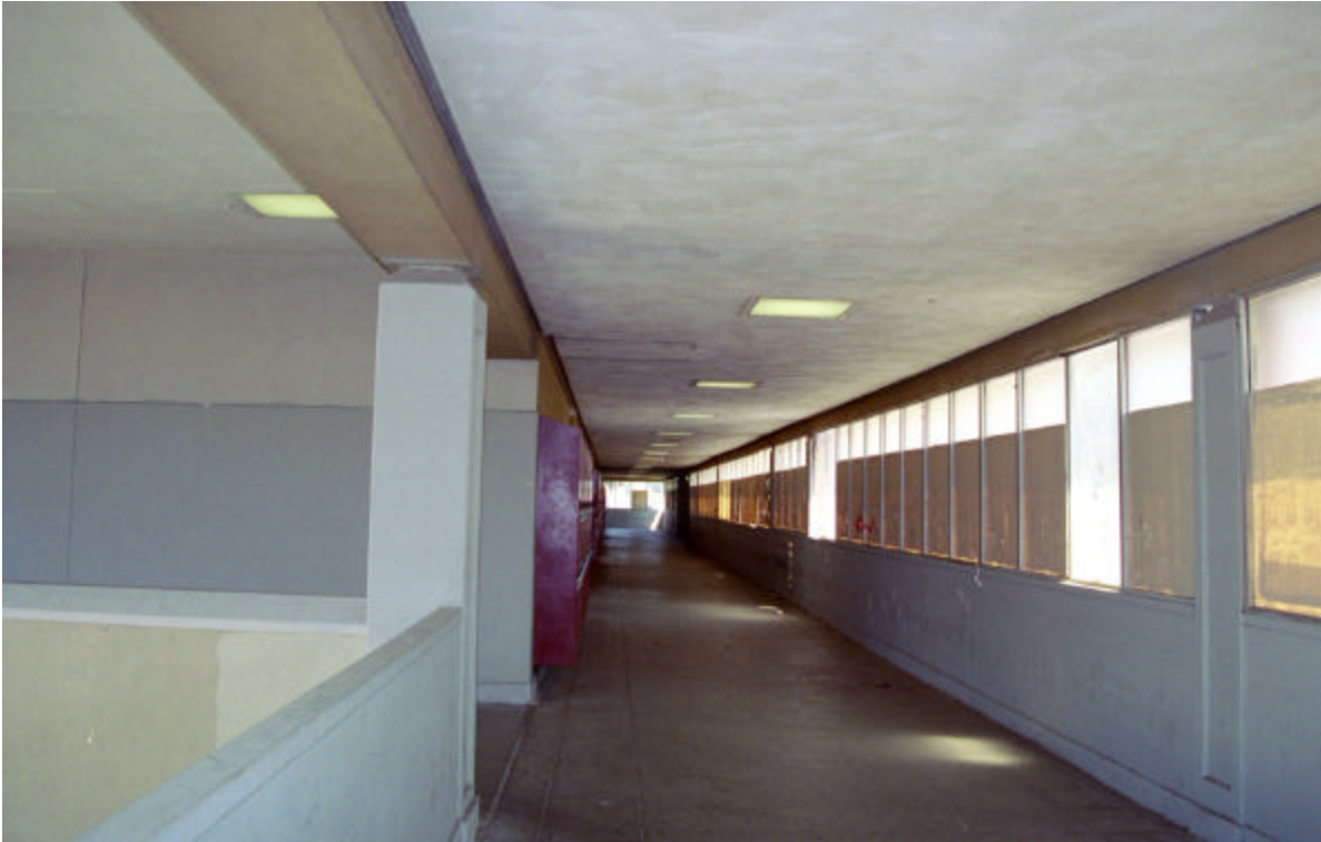
Figure 6: Building 1 Second Floor Corridor
