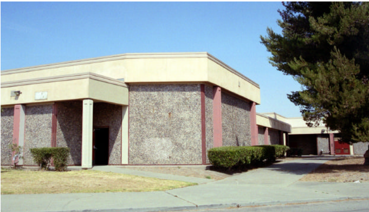
Figure 13: South West Elevation of Theater Building
