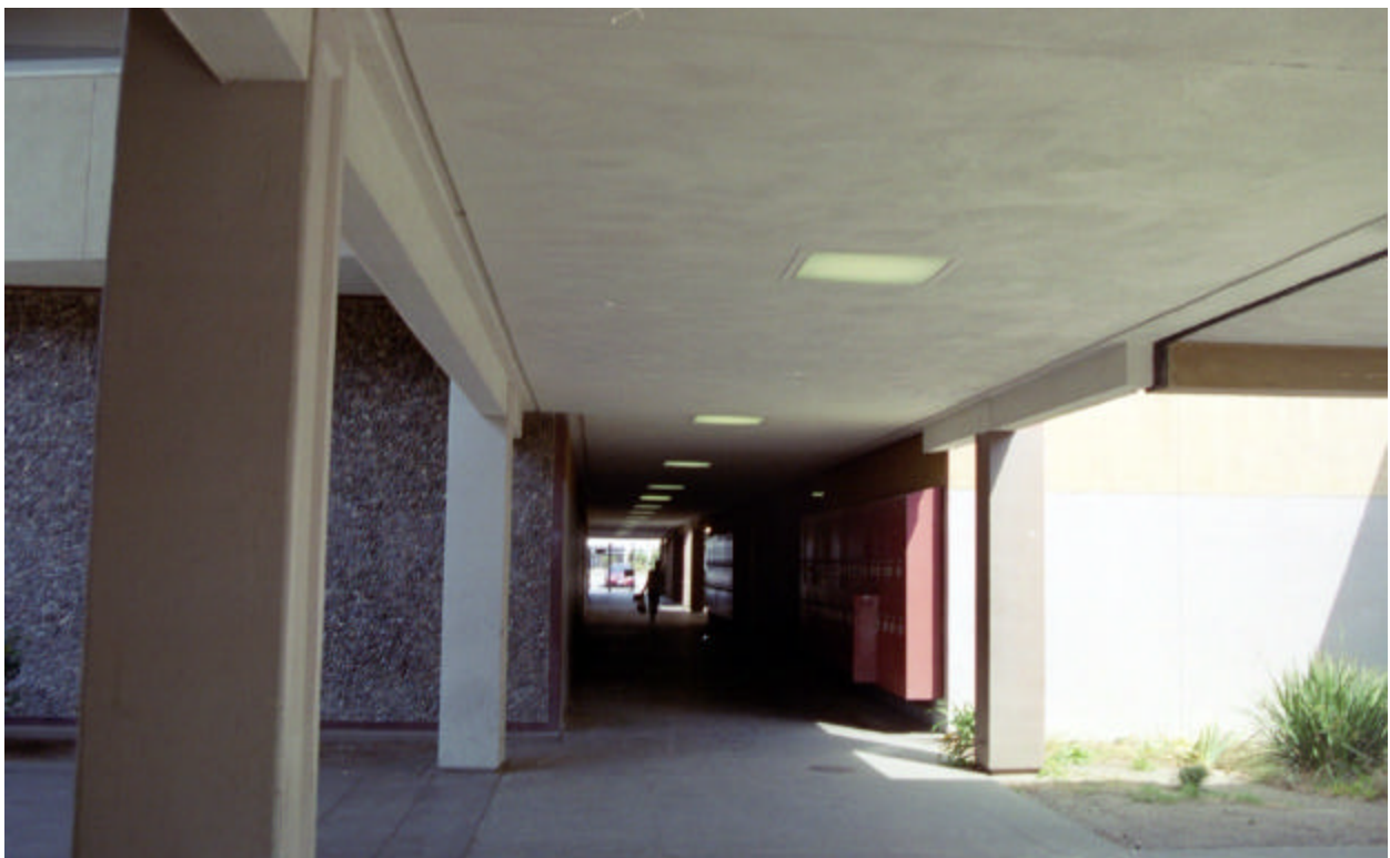
Figure 15: Covered Walkway Connecting Buildings 1 & 11
