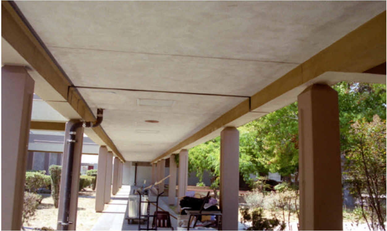
Figure 14: Typical Covered Walkway with Seismic Joint
