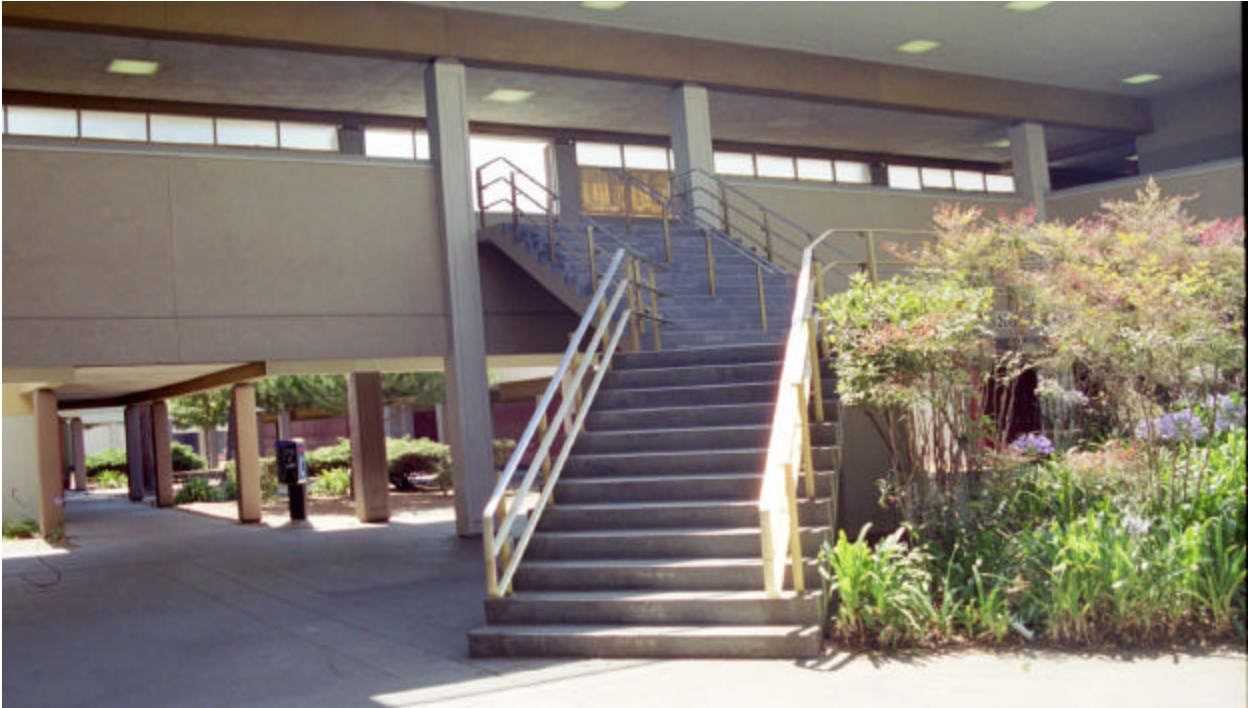
Figure 5: Main Entrance Lobby.
