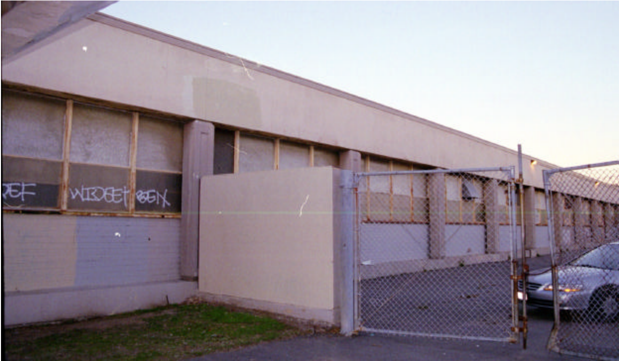
Figure 8: South Wall of Building IV
