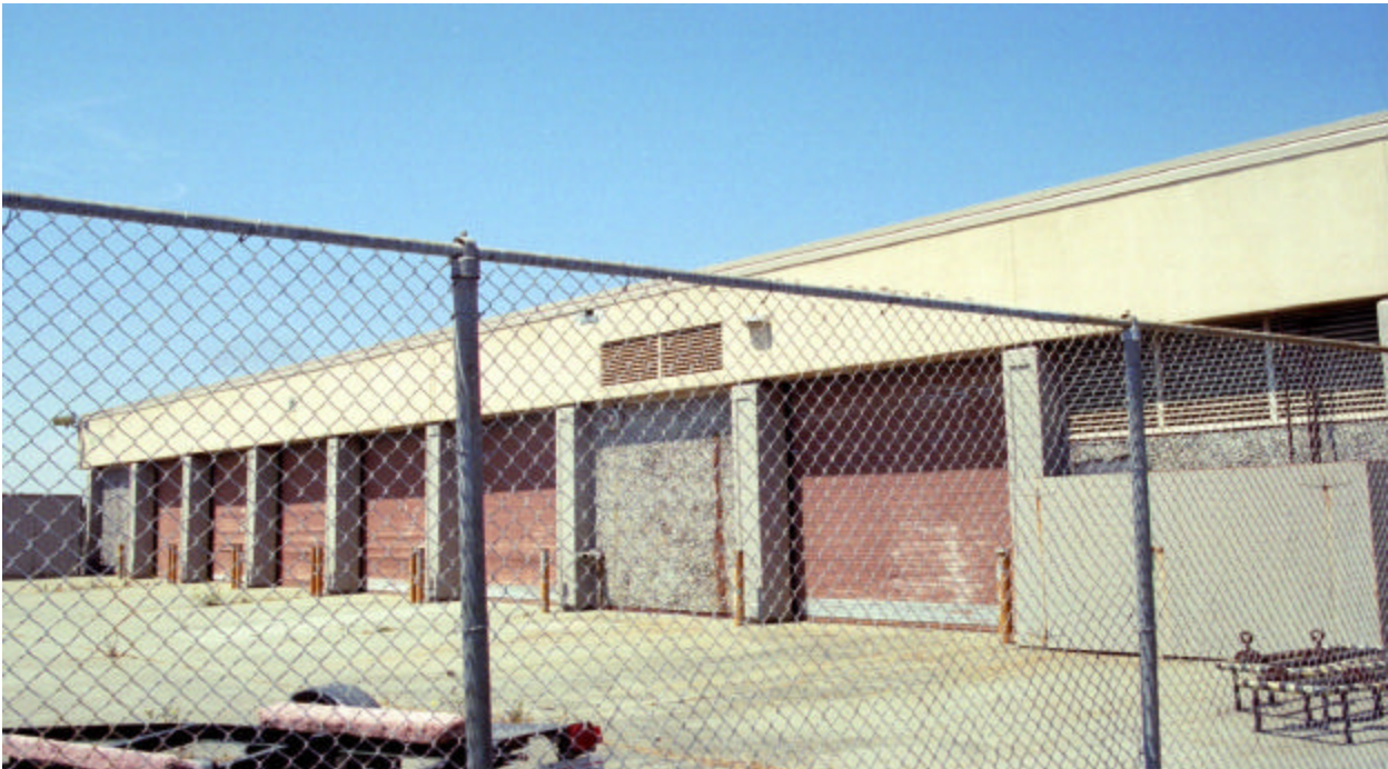
Figure 11: South Wall of Industrial Arts Building
