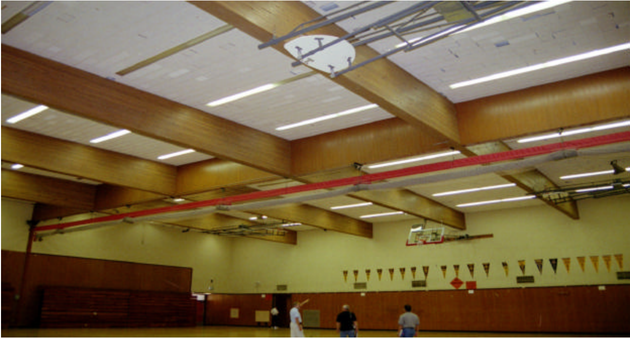
Figure 10: Gymnasium Building Roof Framing
