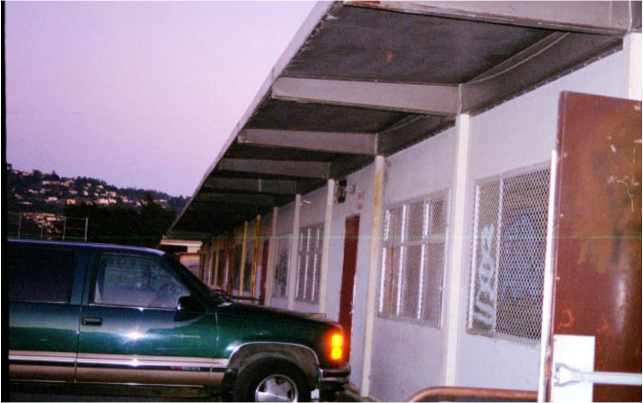
Figure 16: Exterior Wall of Portable Building
