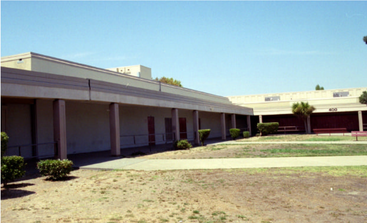
Figure 7: West Elevation of Building IV
